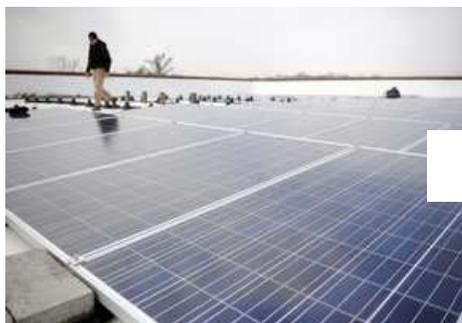
The track system for the panels isn't bolted into the roof surface, but is held down with concrete pavers supplied by OK Coal and Concrete of South Zanesville.
