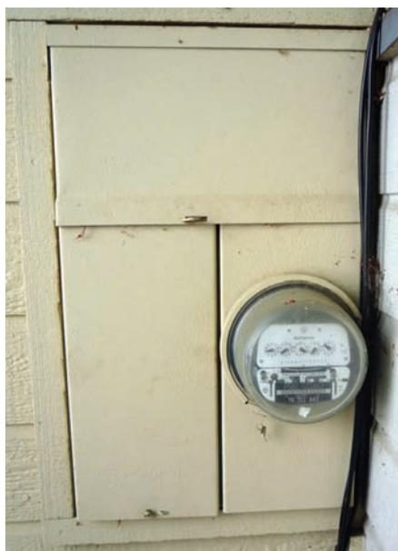
**Figure 1** The sealed portion (lower left) of this all-in-one service entrance device houses the utility’s service lateral, which comes in underground and feeds the meter portion of the device (lower right). The top portion of the device is the distribution panel.
