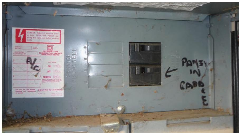
**Figure 2** Opening the cover of the distribution panel reveals a stamped dead plate cover identifying any installed breakers as service disconnecting means.
